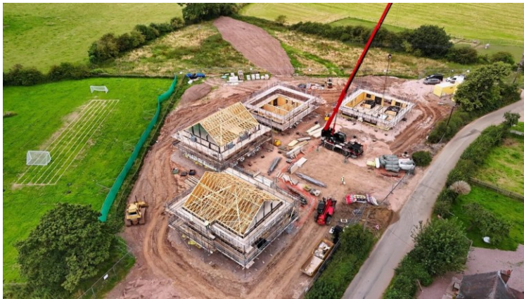
New houses under construction in Bednall - Stafford Aerial Footage Facebook group - Andrew Drone Bird
